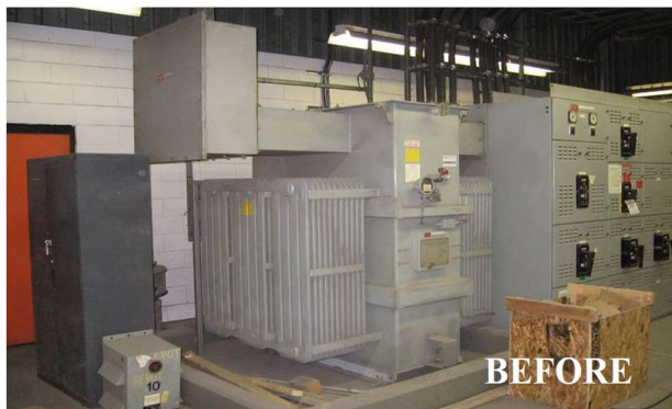
Figure 5: Existing oil type transformer updated by a dry type equivalent 3 000kVA, Montreal airport QC 2009.
